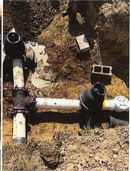
Figure 3: New drain valves at splash pad
