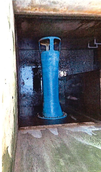
Figure 2: Remove chlorine diffuser
