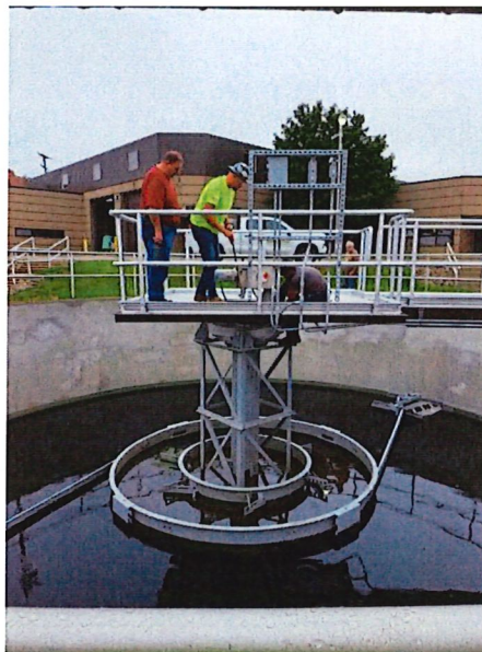
Figure 5: Repairs to Clarifier
