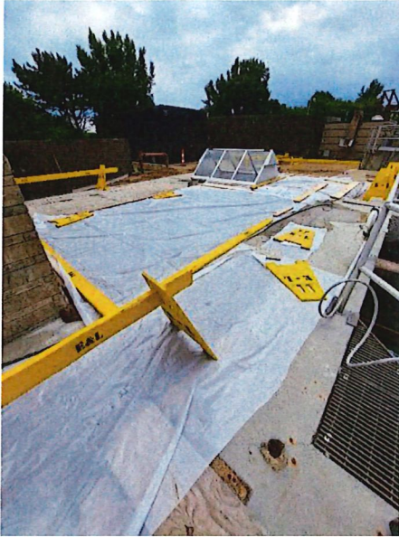
Figure 1: New concrete deck
